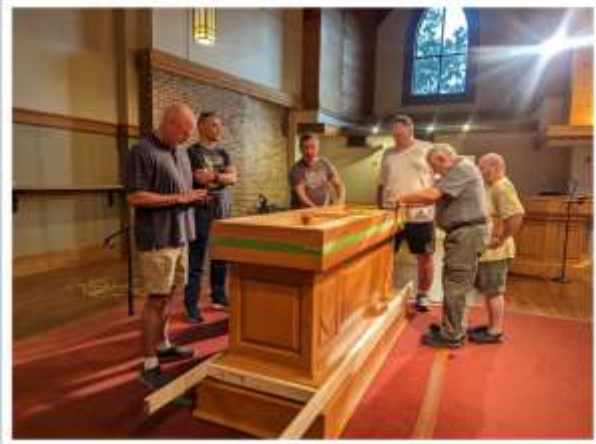
Below: A dedicated team of Handy-MoMs led by Richard Webb, gathered on May 9 to reduce the height of the altar to make it more comfortable for Pastor Kris and Altar Guild members. Once it was cut down, the team came back and added quarter-round wooden moulding to finish the look. Great job team! We now can see our new pastor much better during worship!
